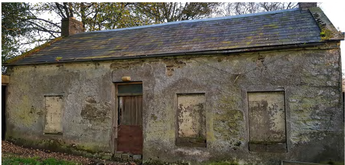
Photo 15 – Building A front view.
