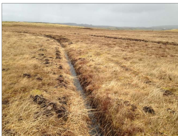
Plate 4. Cleaned out drainage ditches east of T3
