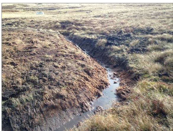
Plate 3. Recently cleaned drainage ditch at T4
