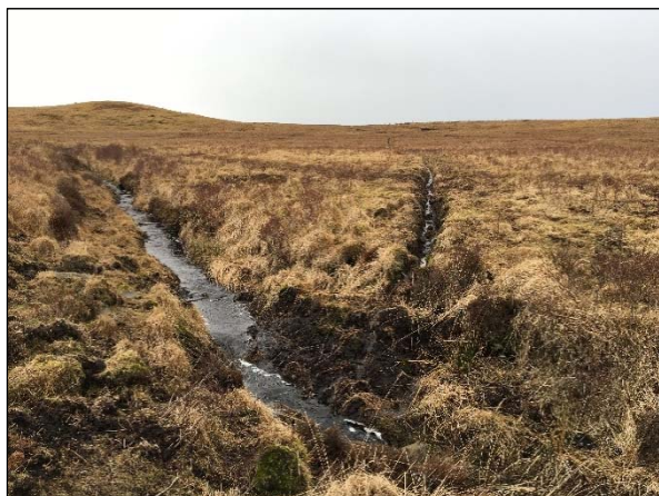
Plate 1. Drainage ditches at T3 cleaned out, with water freely flowing.
