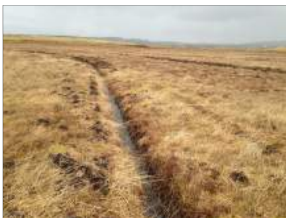
Plate 4. Cleaned out drainage ditches east of T3
