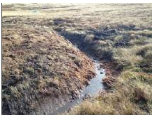
Plate 3. Recently cleaned drainage ditch at T4
