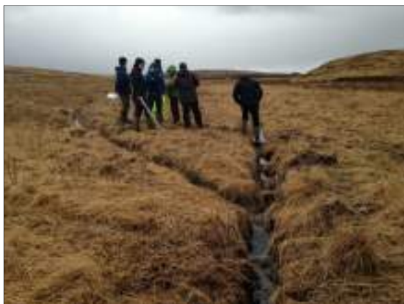
Plate 1. Drainage ditches at T3 cleaned out
