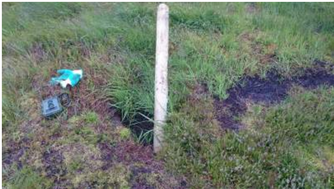
Plate 5 - The collapsed tunnel at 54745 11466 (bottom of post) with gloves and trail camera for scale.
