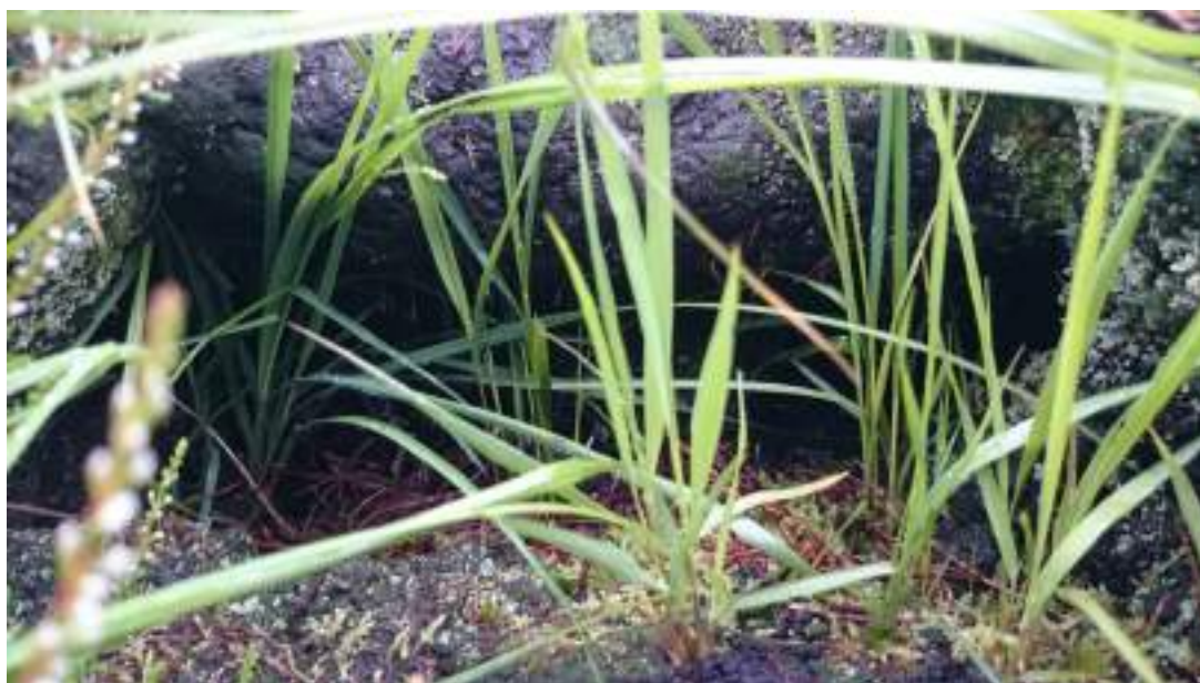
Plate 6 - A close-up of the collapsed tunnel entrance showing grass and the lack of obvious signs of any recent use of the tunnel/burrow/den/sett.
